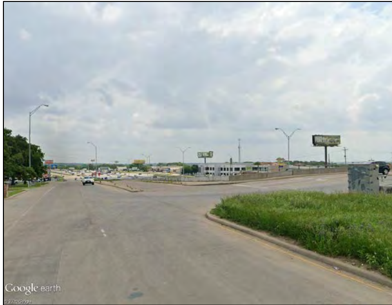
Photo ID 13: View of two-way frontage road and Anglin Drive, facing east.
