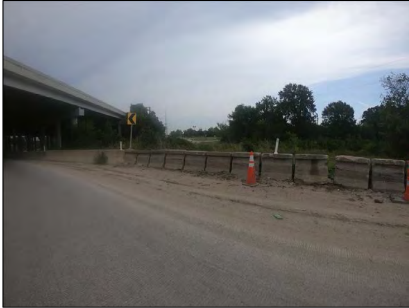
Photo ID 11: View of eastbound I-20 frontage road that ends at UPRR.
