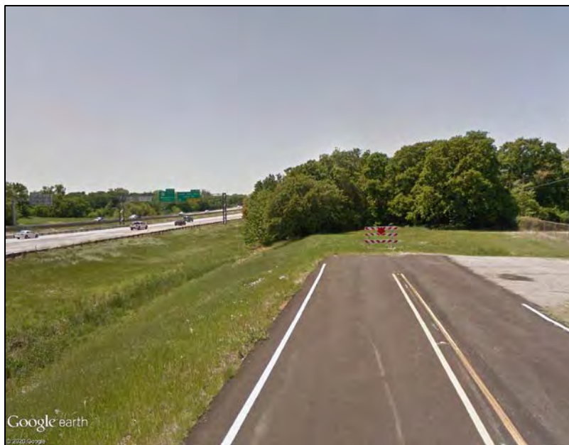
Photo ID 14: View of westbound I-20 frontage road that ends at Kee Branch crossing.
