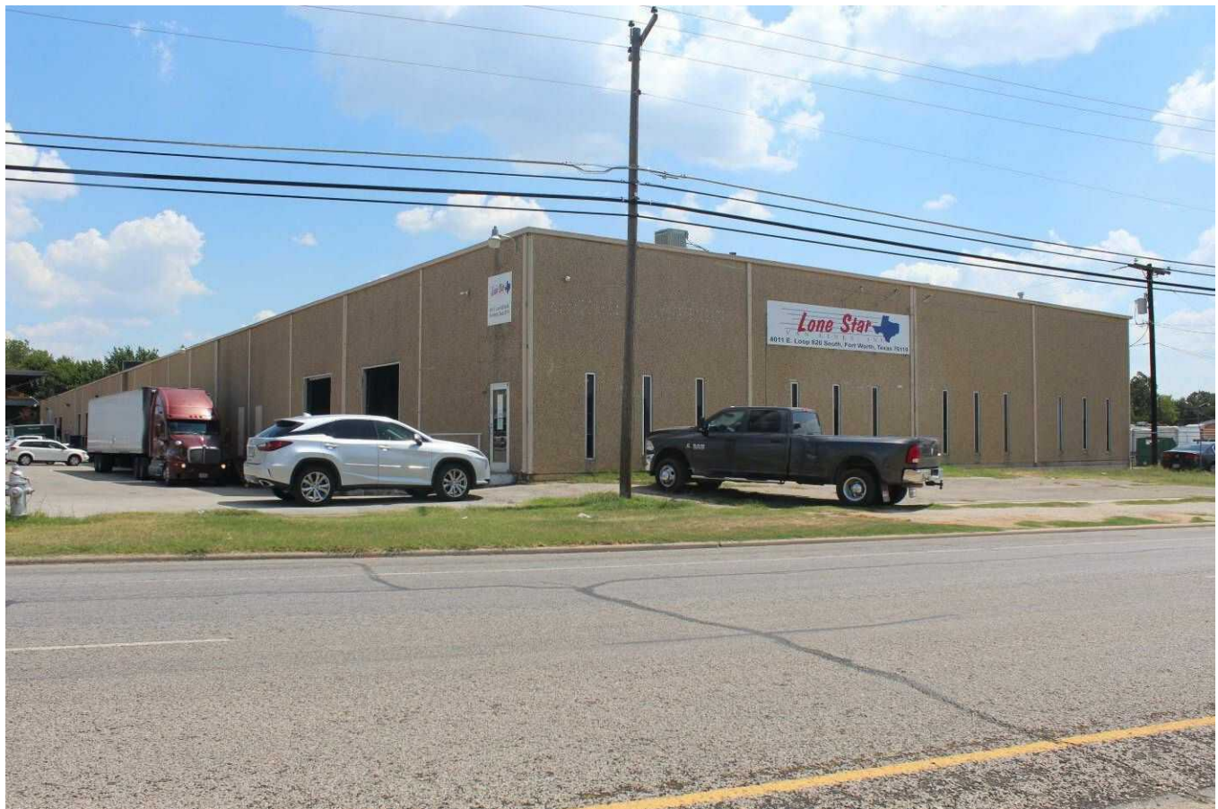
Camera facing east.
