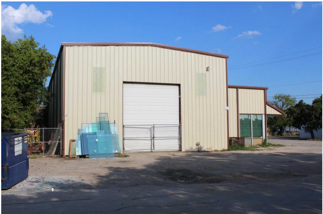
Camera facing east.
