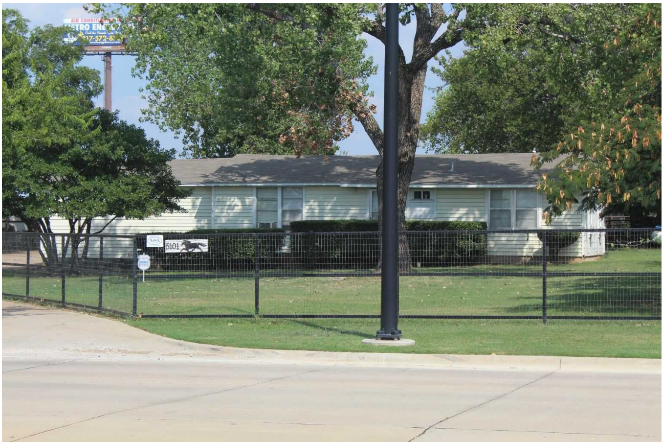
Camera facing east.
