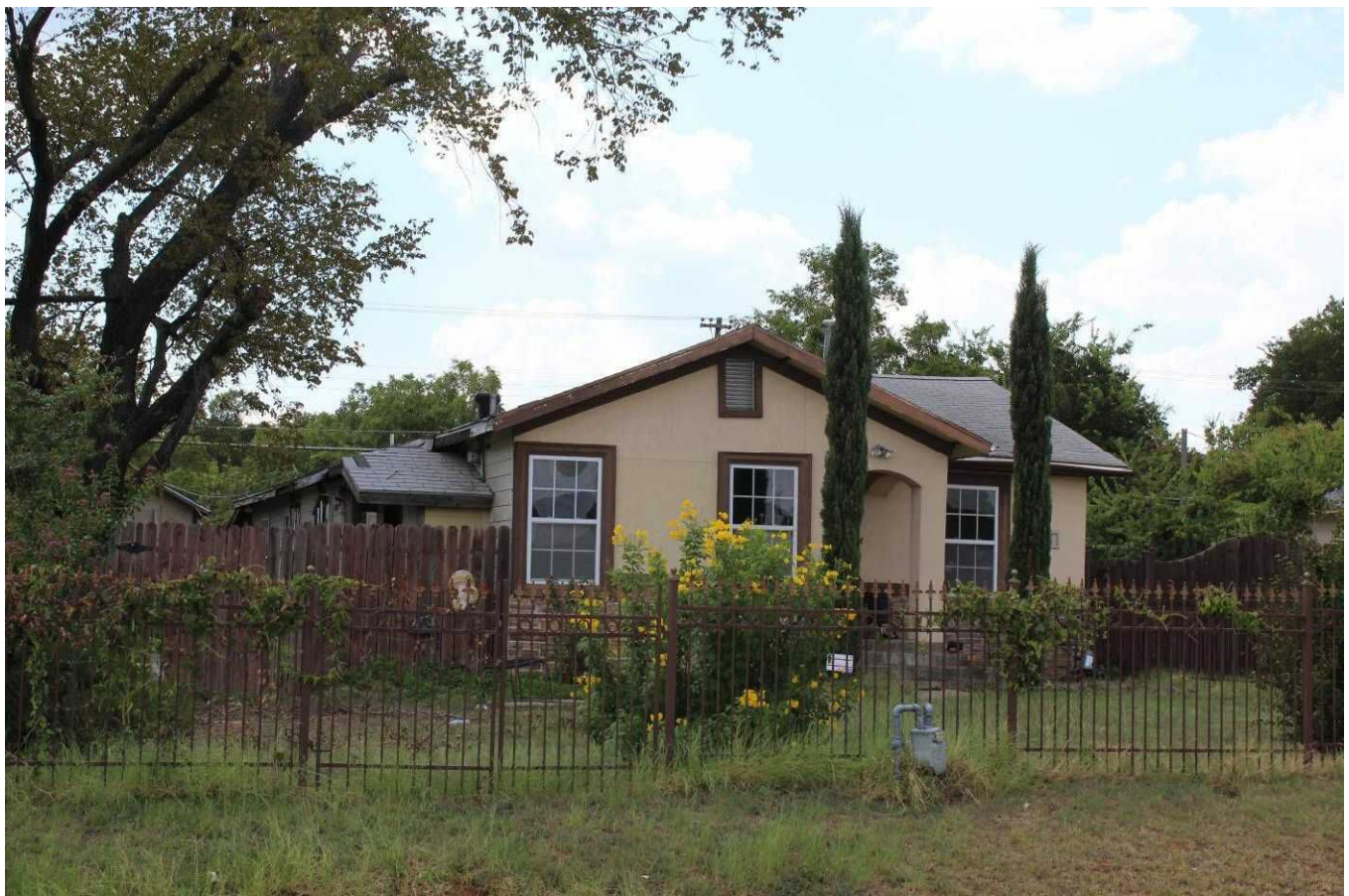
Camera facing west.
