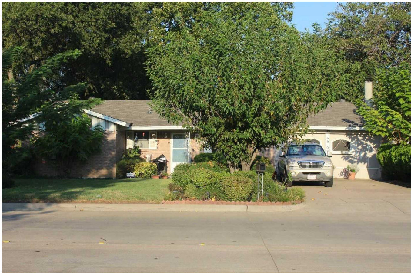
Camera facing west.
