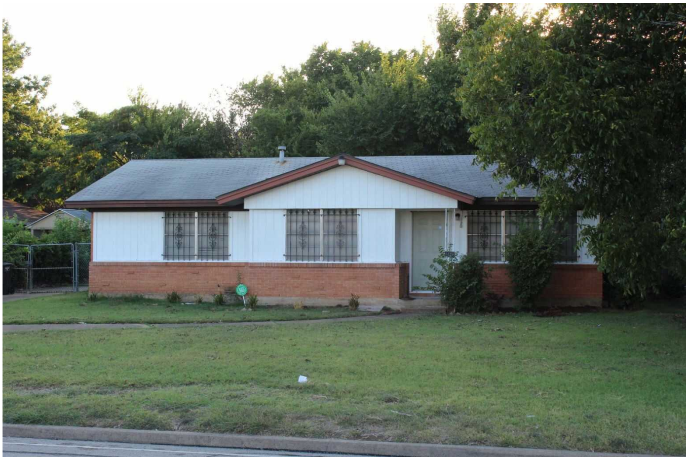
Camera facing west.
