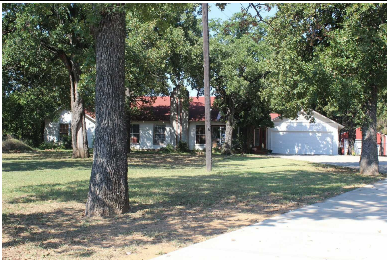
Camera facing west.
