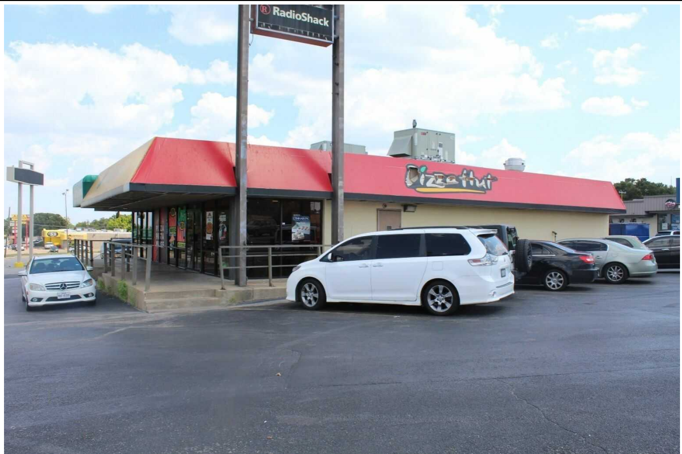
Camera facing east.
