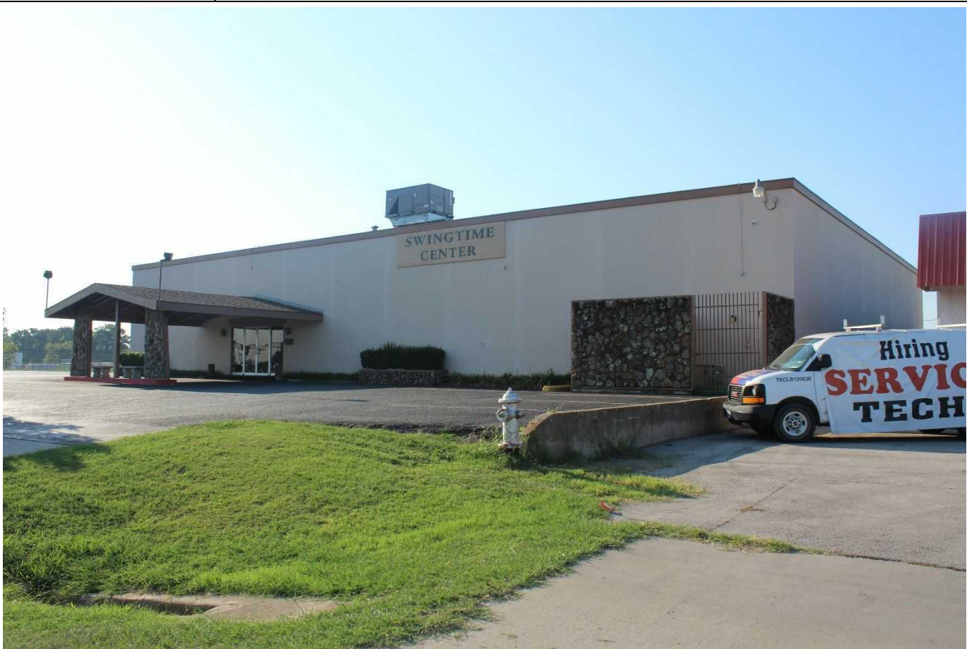
Camera facing southeast.
