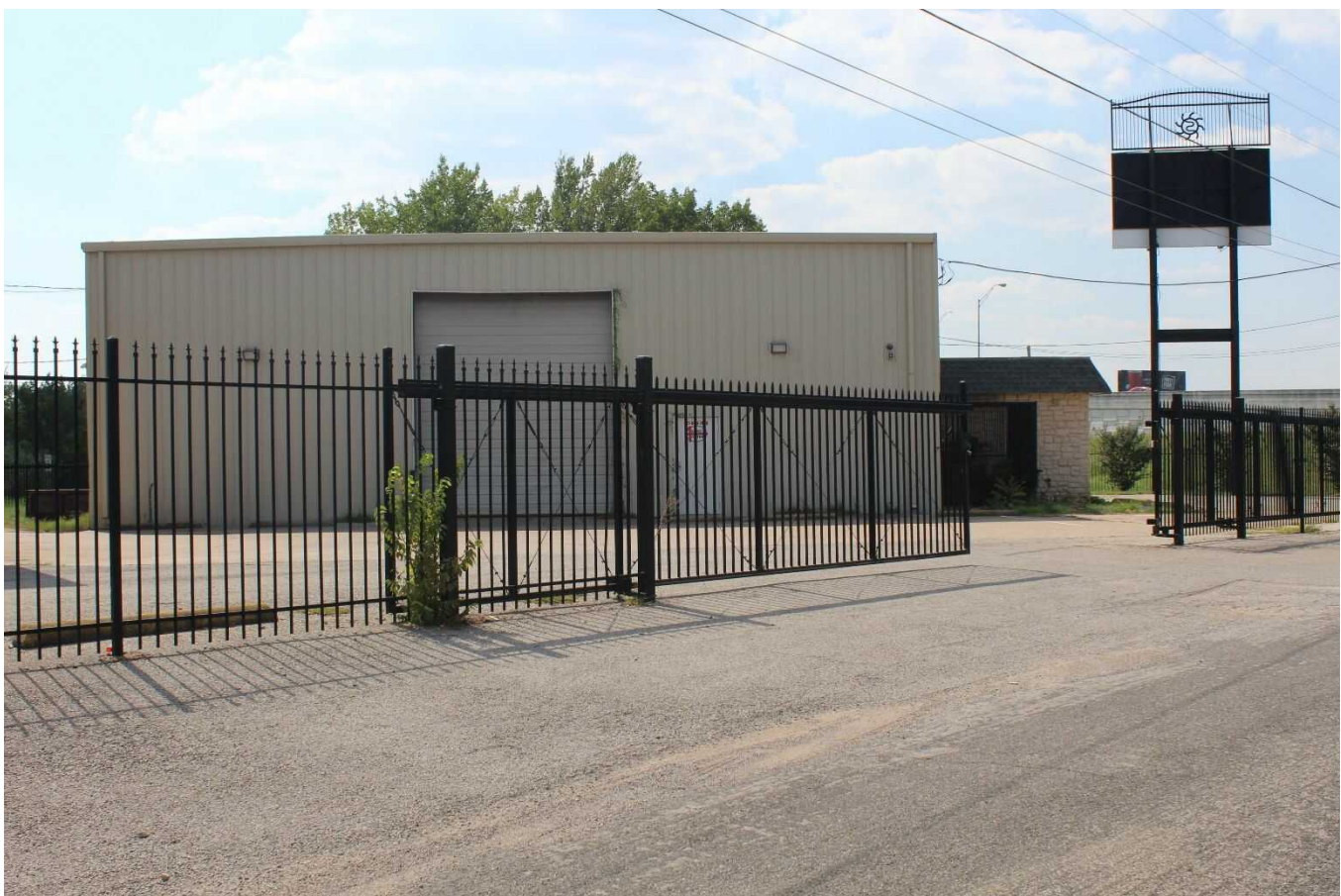
Camera facing west.
