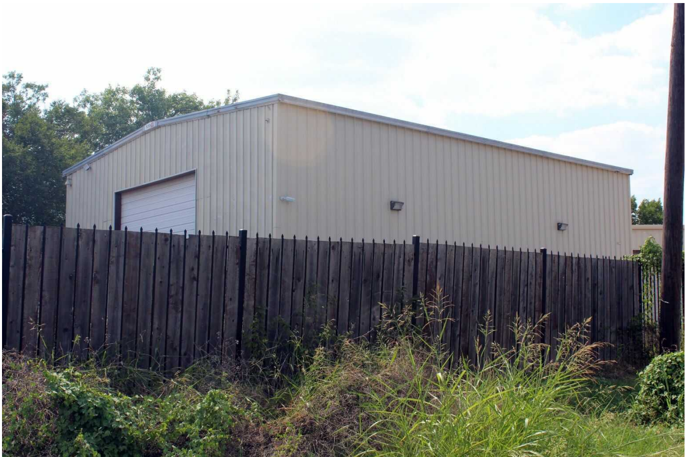
Camera facing west.
