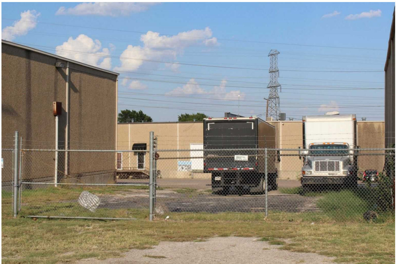
Camera facing east.
