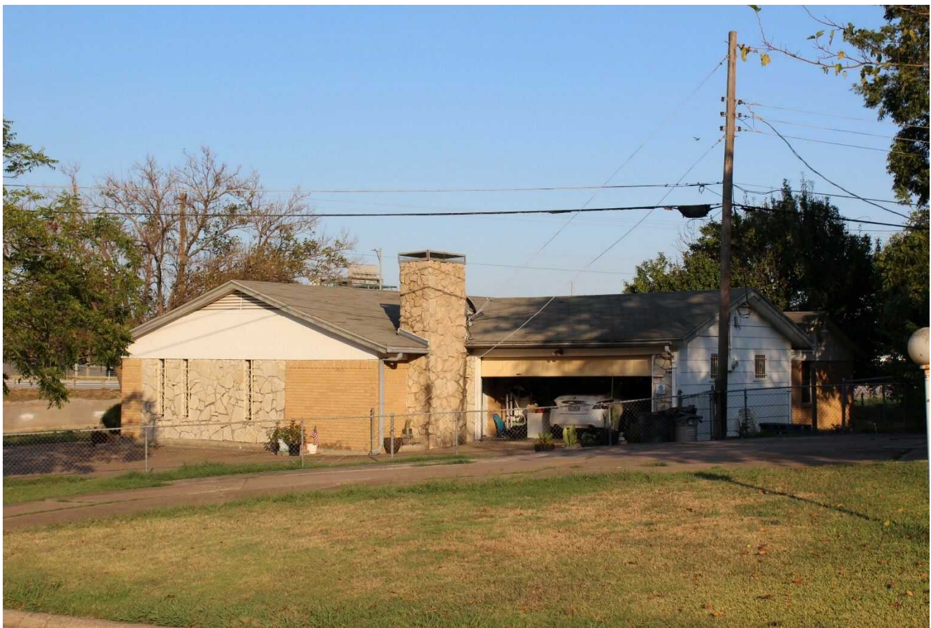
Camera facing east.
