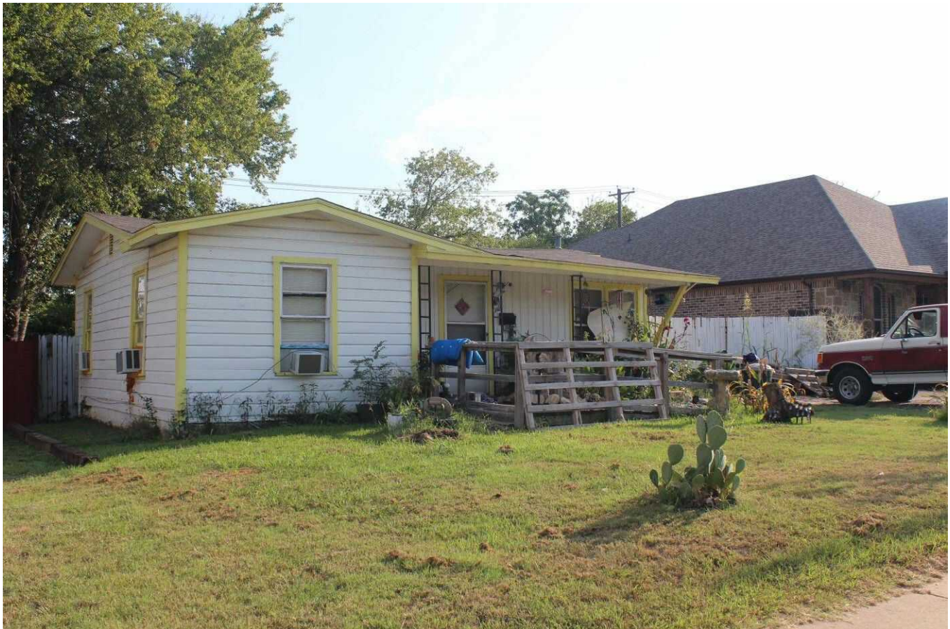
Camera facing west.
