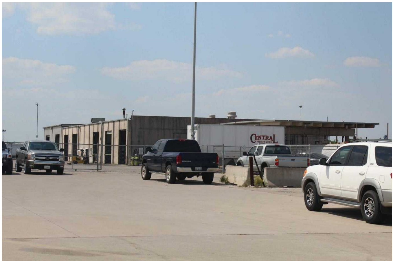
Camera facing west.
