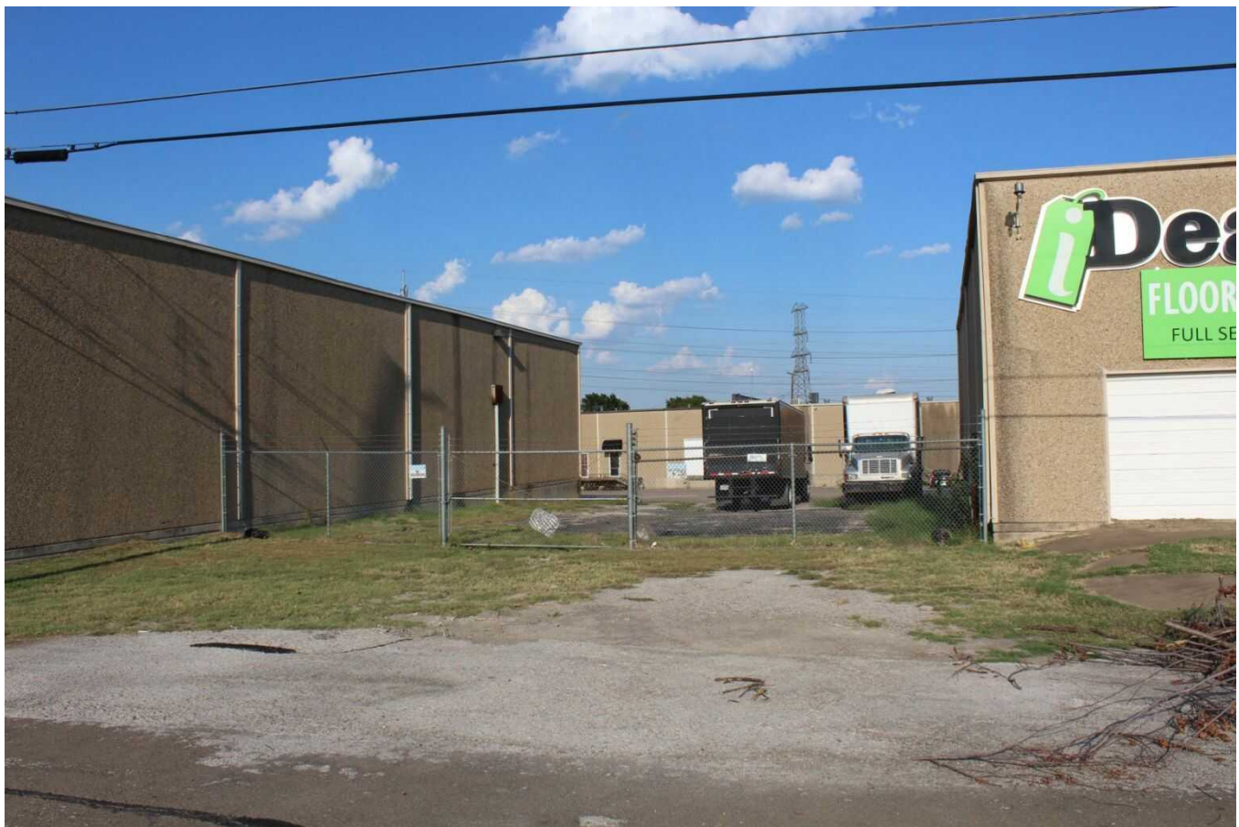
Camera facing east.
