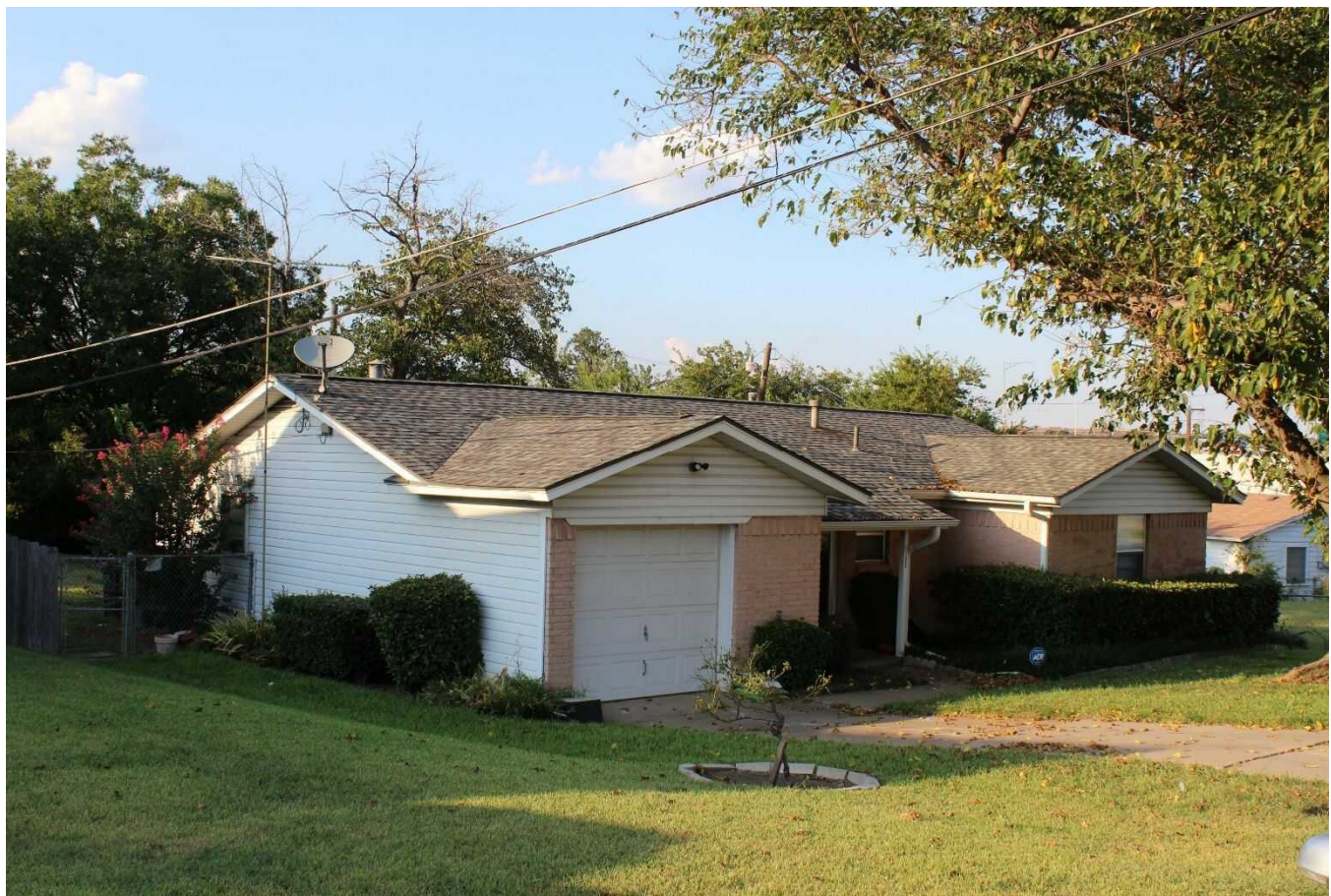
Camera facing east.
