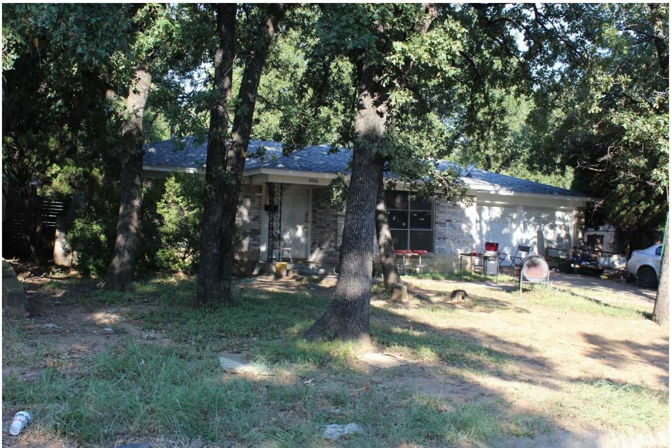
Camera facing west.
