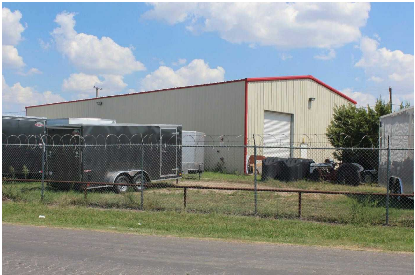
Camera facing east.
