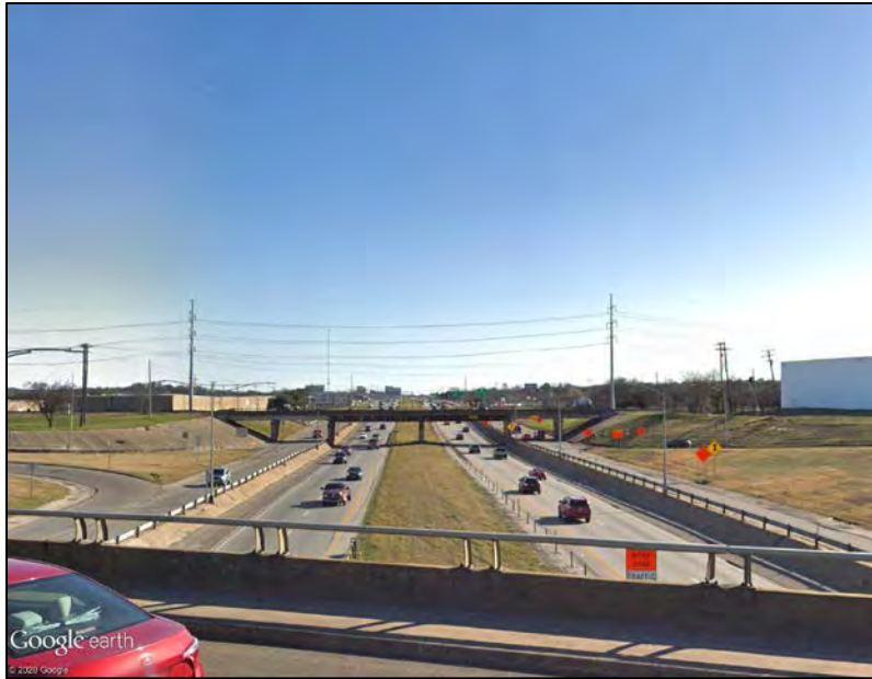
Photo ID 9: View of I-820 looking south from East Lancaster Avenue.
