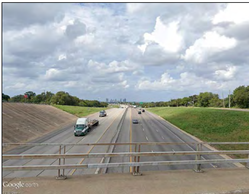
Photo ID 4: View of US 287 looking northwest from Erath Street.
