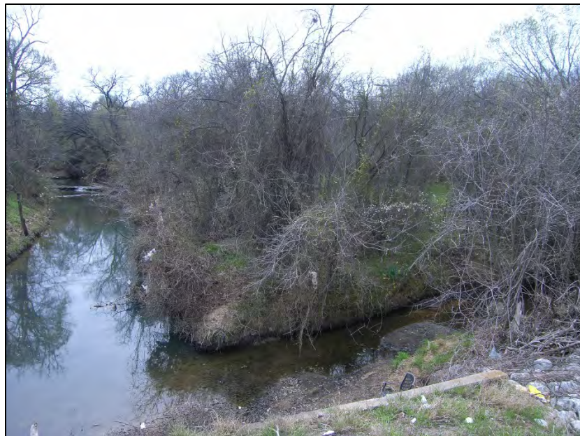
Photo ID 18: View of Crossing 5, Kee Branch and confluence with a tributary south of eastbound I-20 main lanes.
