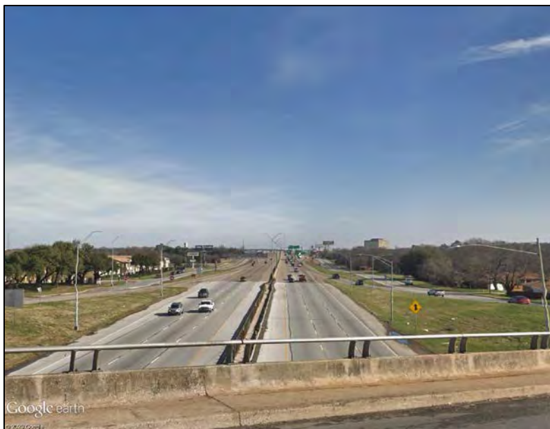
Photo ID 10: View of I-820 looking north from Meadowbrook Drive.
