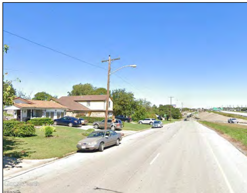
Photo ID 16: View of Carver Heights Historic District (left) located adjacent to southbound I-820 frontage road looking north.
