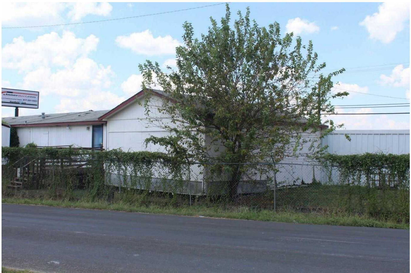
Camera facing west.
