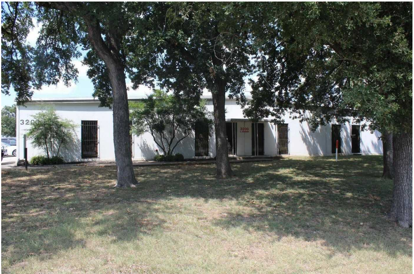
Camera facing west.
