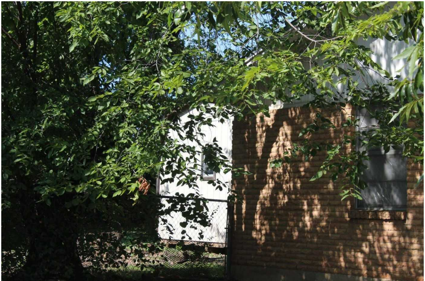
Camera facing west.
