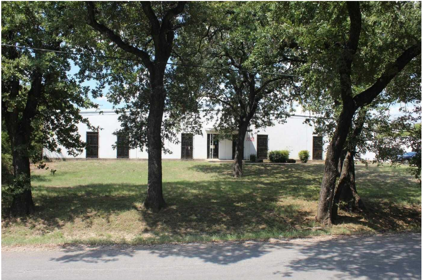
Camera facing west.
