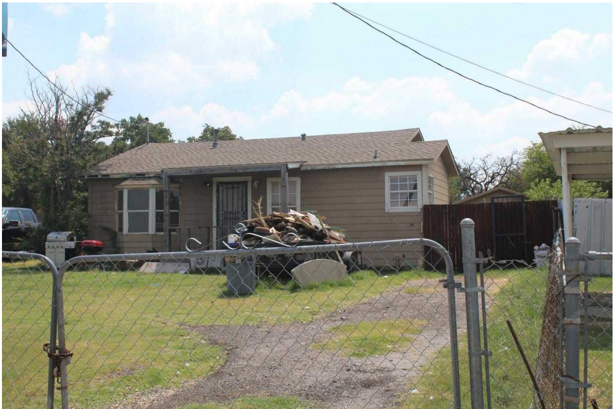
Camera facing west.
