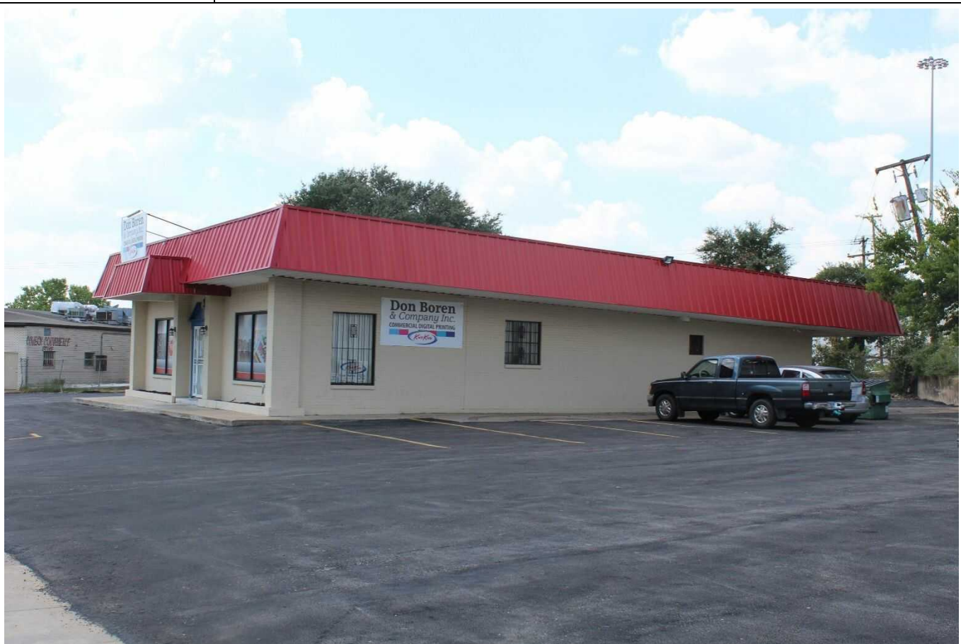
Camera facing west.
