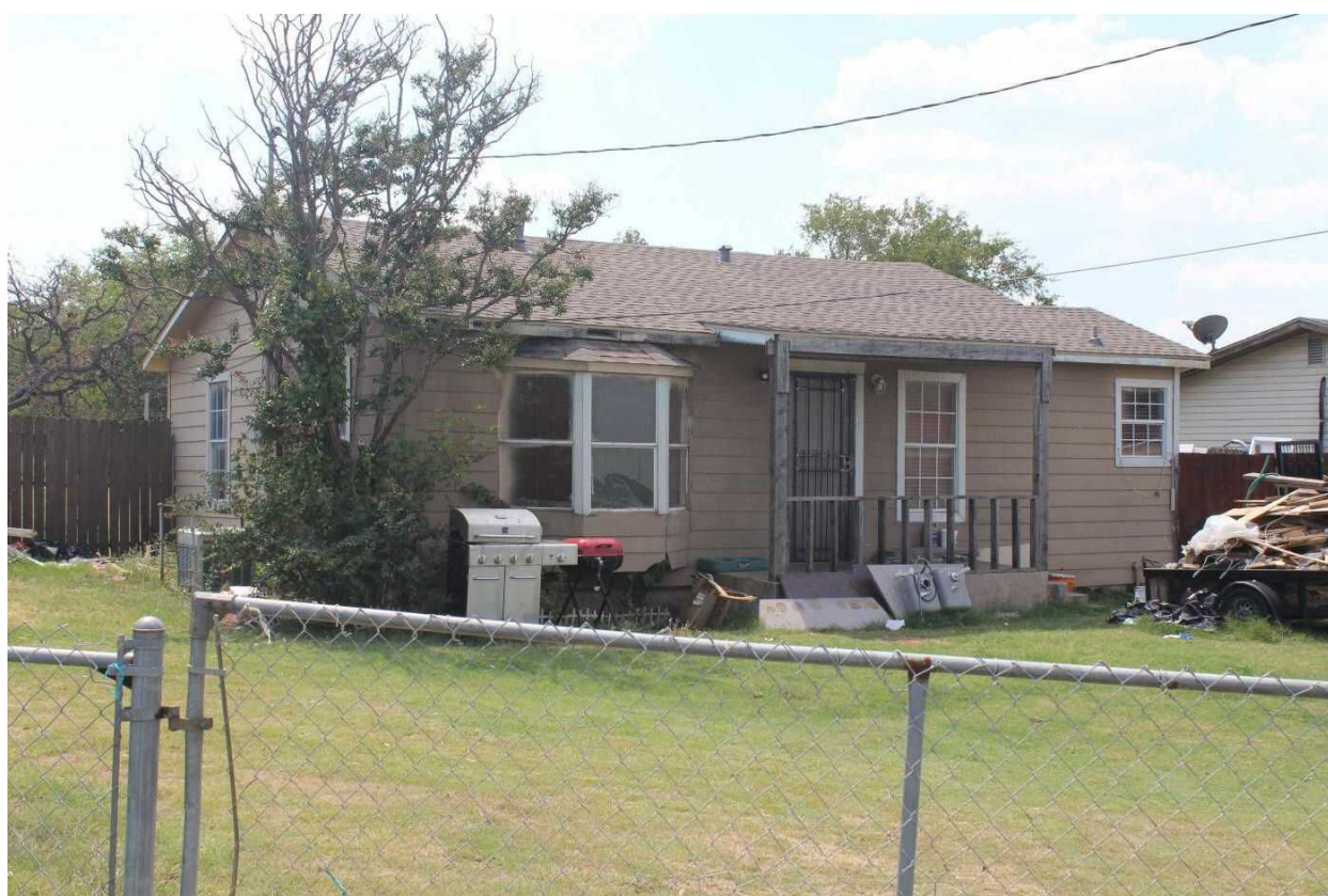
Camera facing west.
