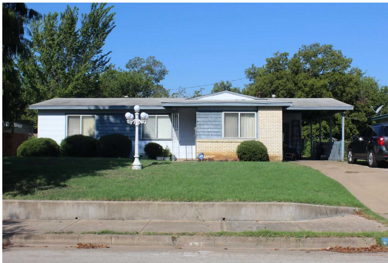
Camera facing west.
