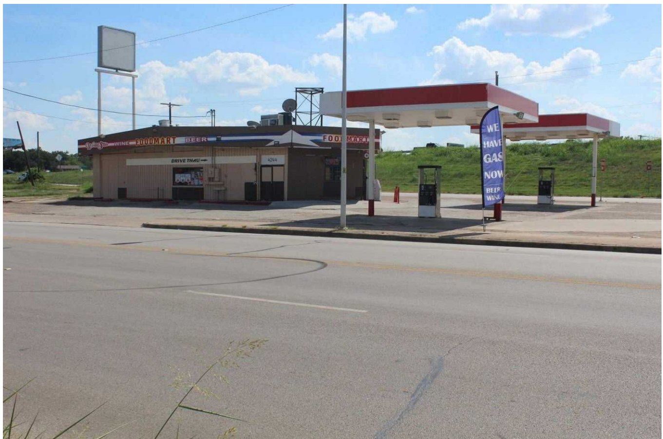
Camera facing west.
