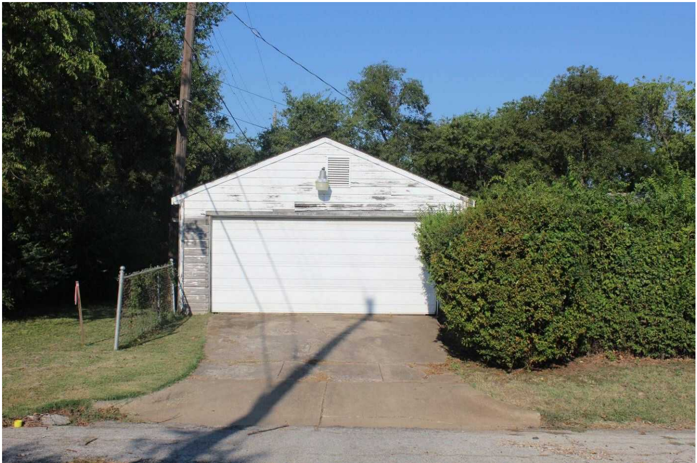
Camera facing west.
