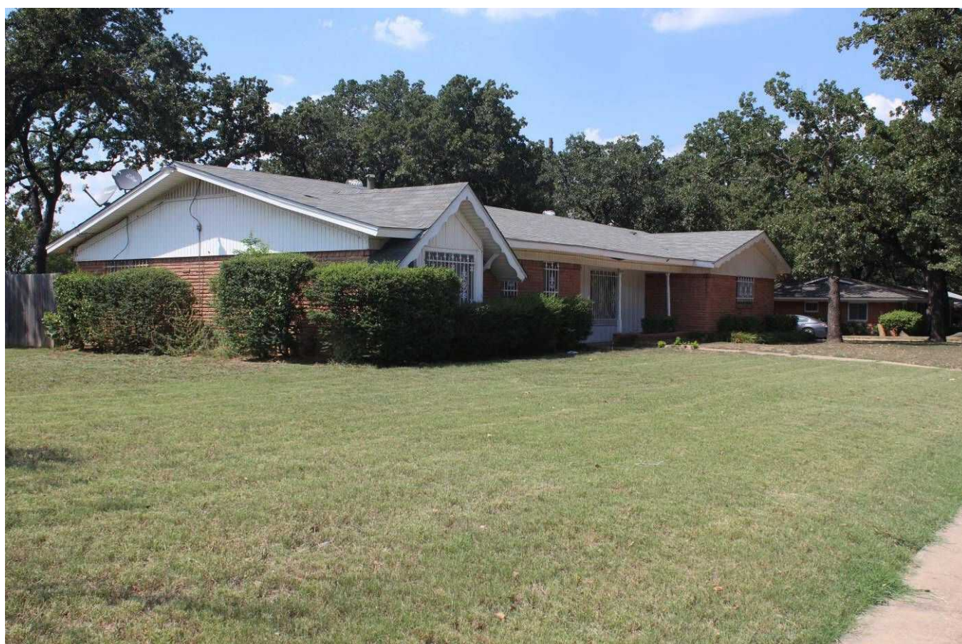
Camera facing west.
