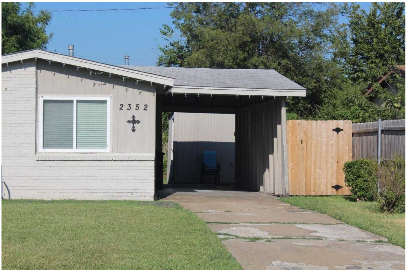
Camera facing west.
