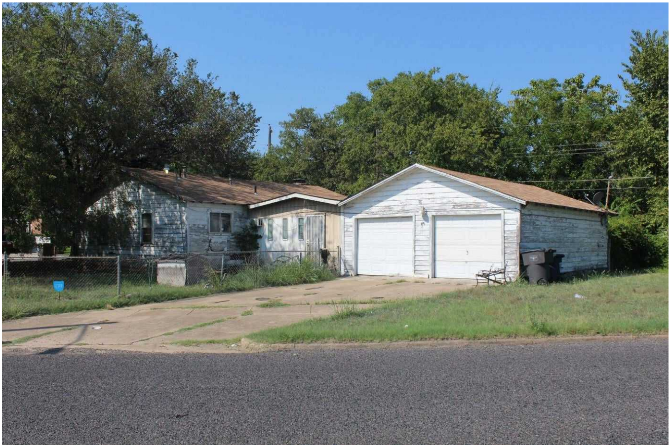
Camera facing west.
