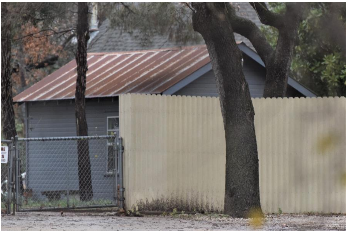
View of non-historic age shed, facing northwest
