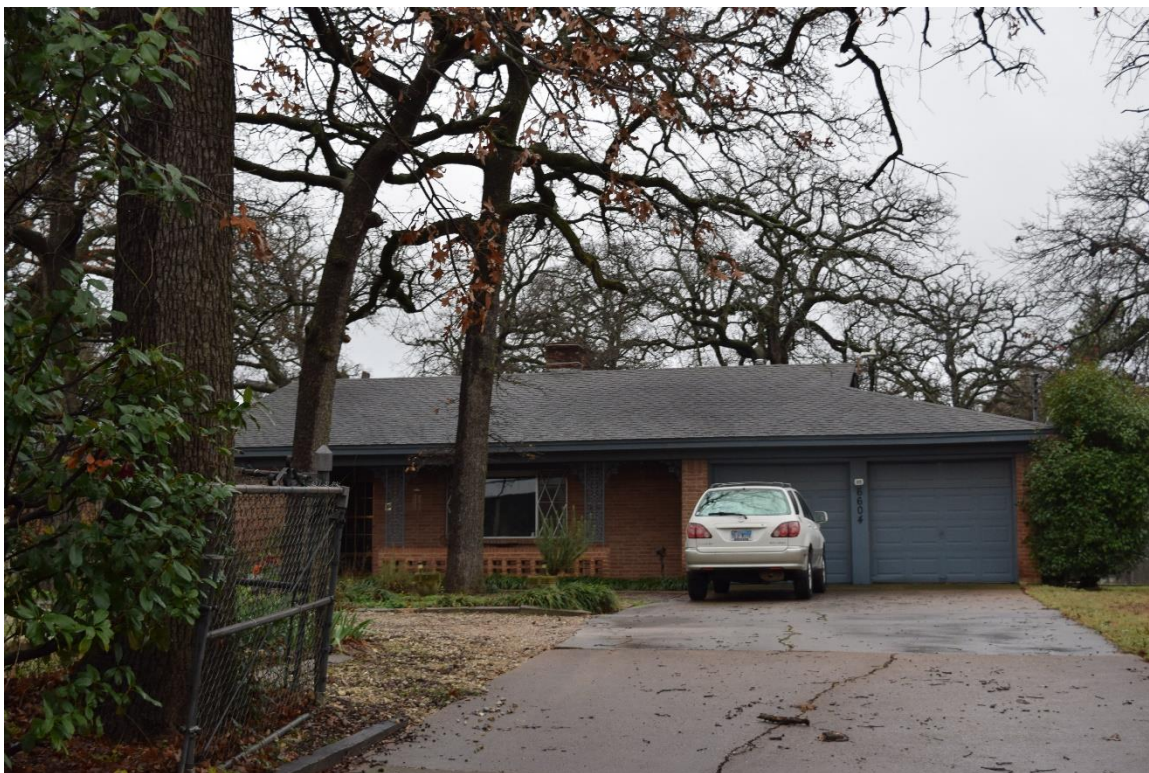
Front elevation facing west
