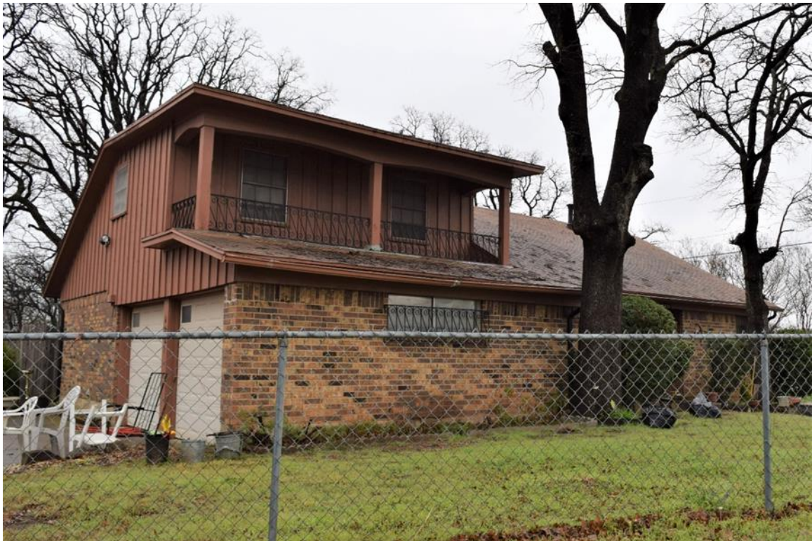
Oblique facing southeast
