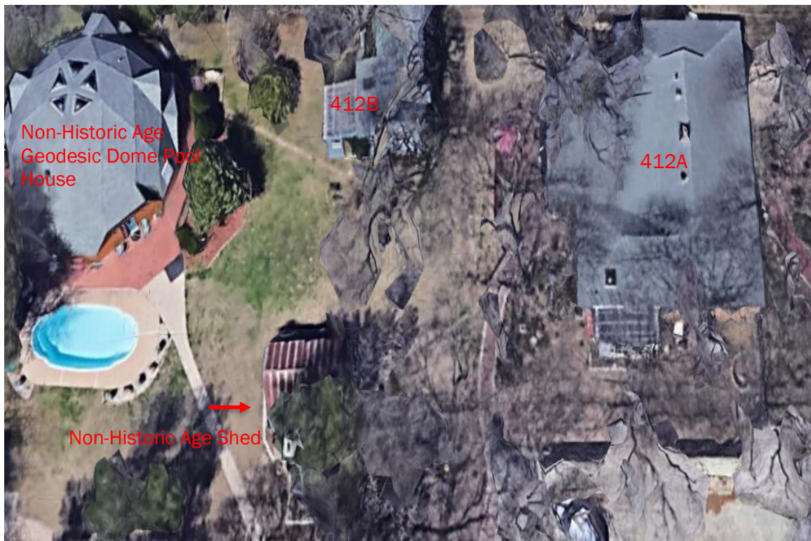
Overview of the proximity of the pool house to Resource Nos. 412A and 412B (image courtesy of Google Earth, 2019)
