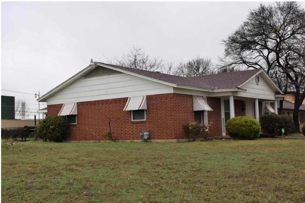
Oblique facing northwest
