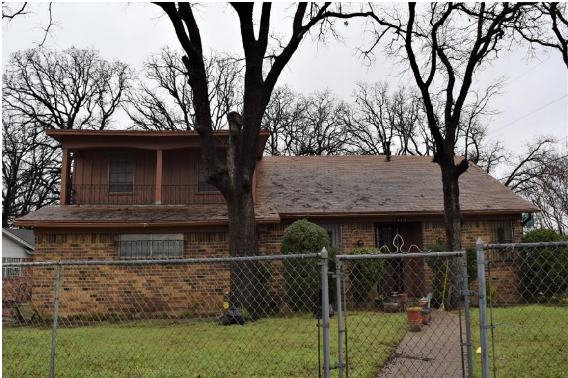
View of front elevation, facing east-southeast
