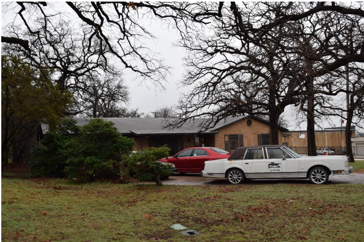
Oblique facing northeast
