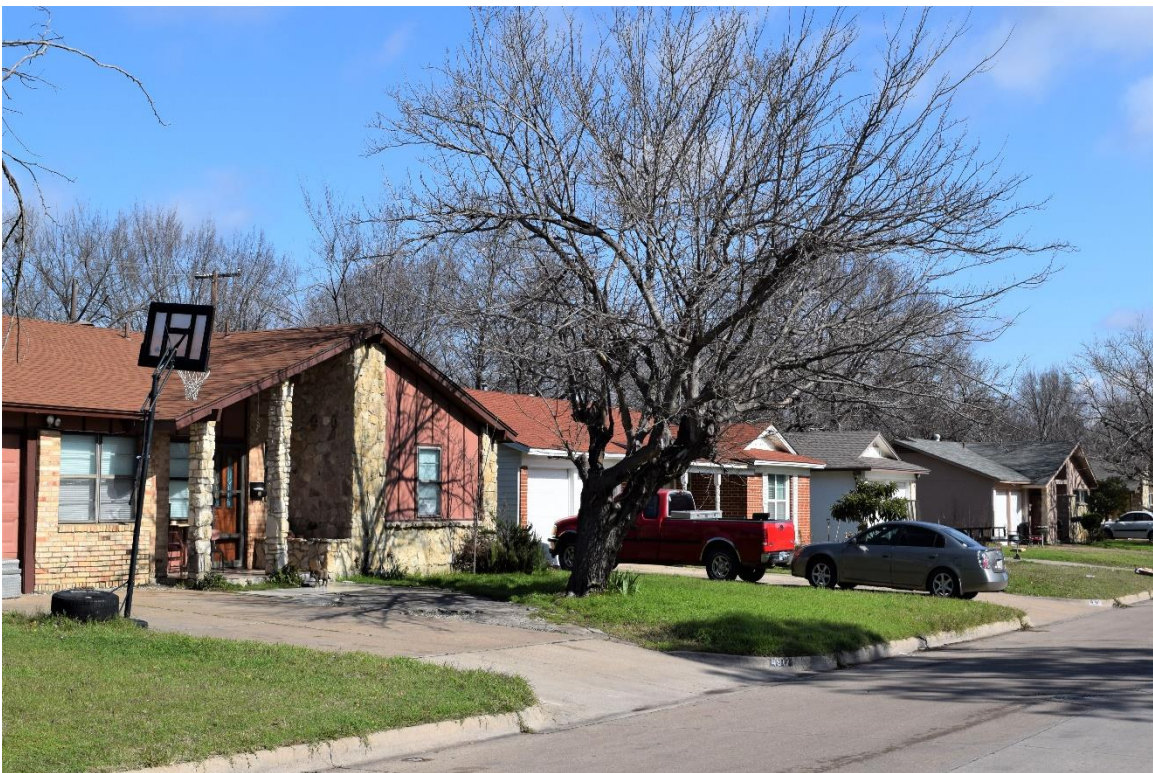
F14: Overview of residences on Suellen Street in Forest Wood Addition (north of Resources No. 432, 435, and 438), facing northeast
