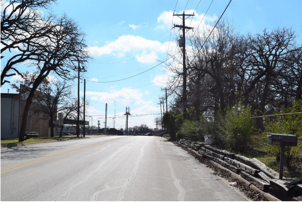
F10: Overview of Anglin Drive, facing south
