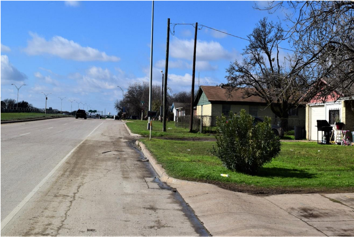
F30: Overview of E. California Parkway, the southern boundary of the Shady Hill Addition (Resource No. 406 on right), facing west
