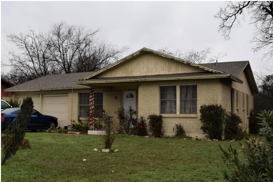
Oblique facing northwest
