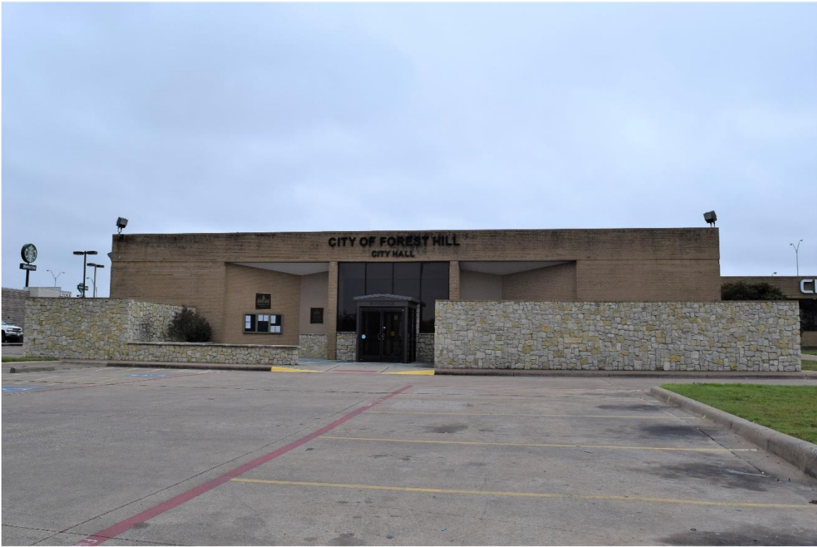
F7: Forest Hill City Hall, facing south
