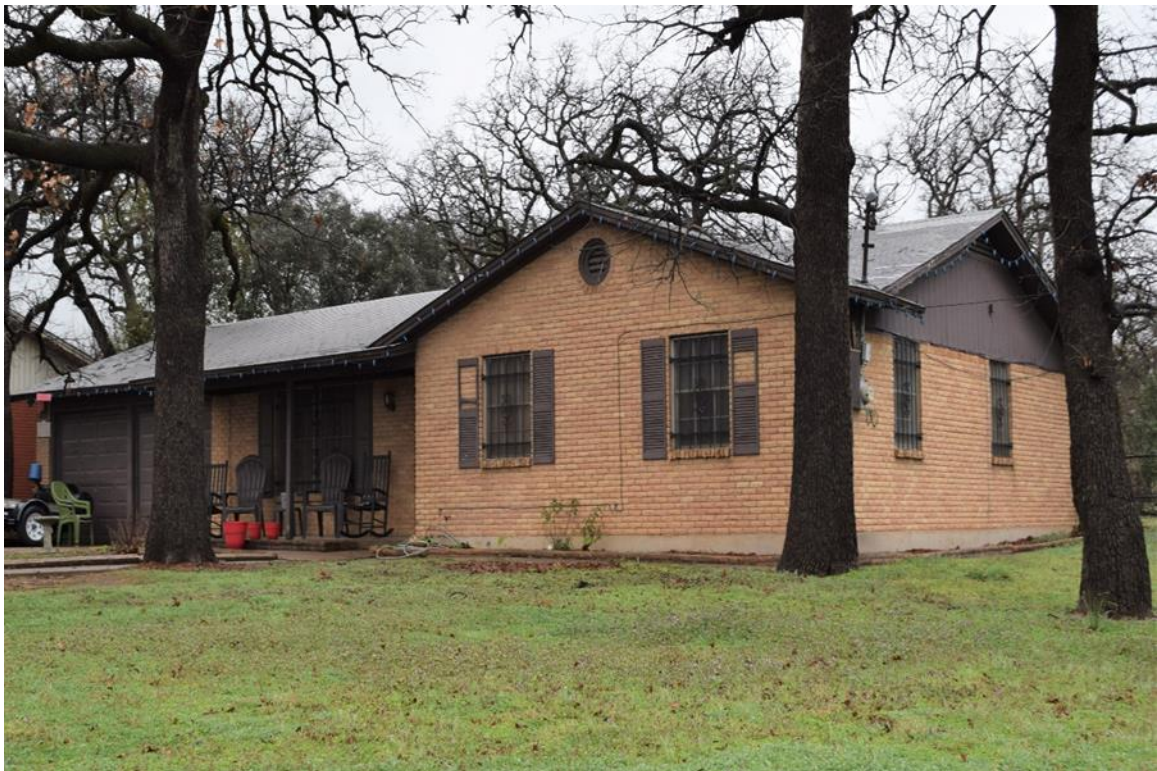
Oblique facing northwest
