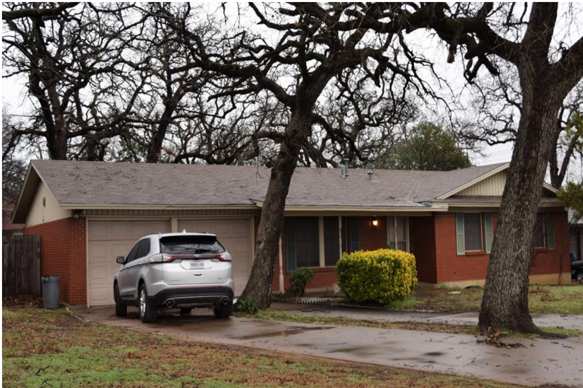
Oblique facing northeast
