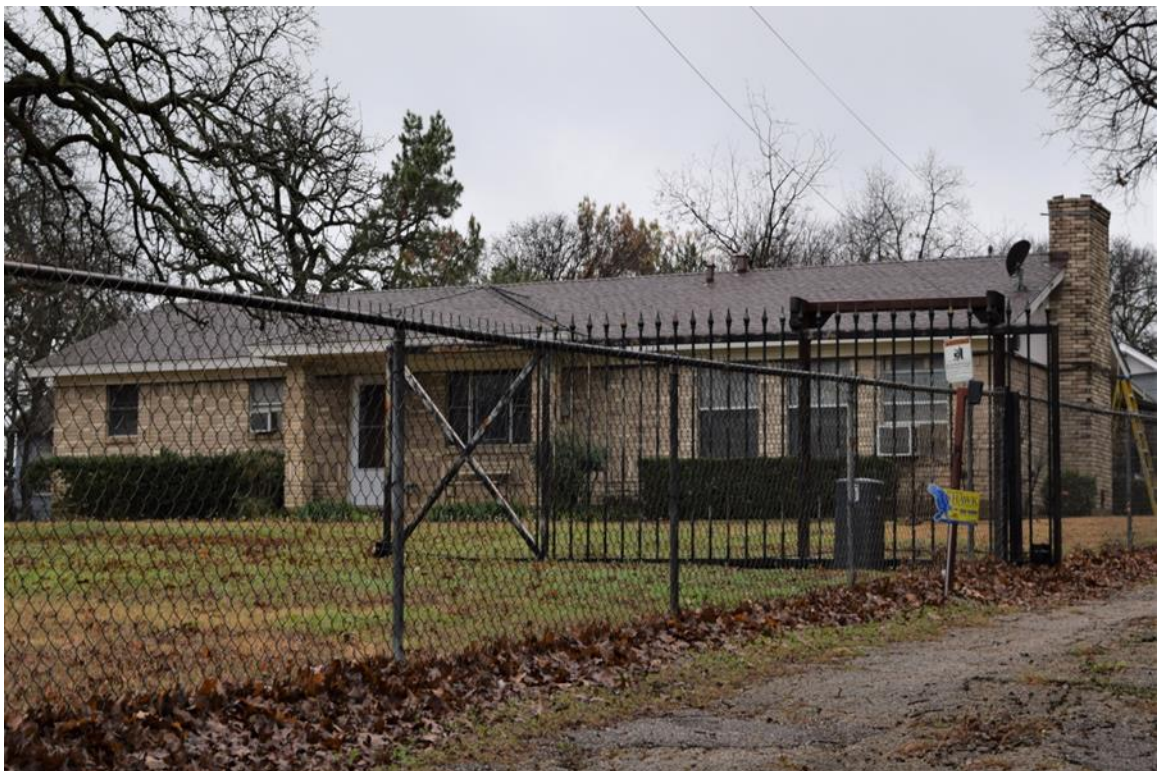
Oblique facing southwest
