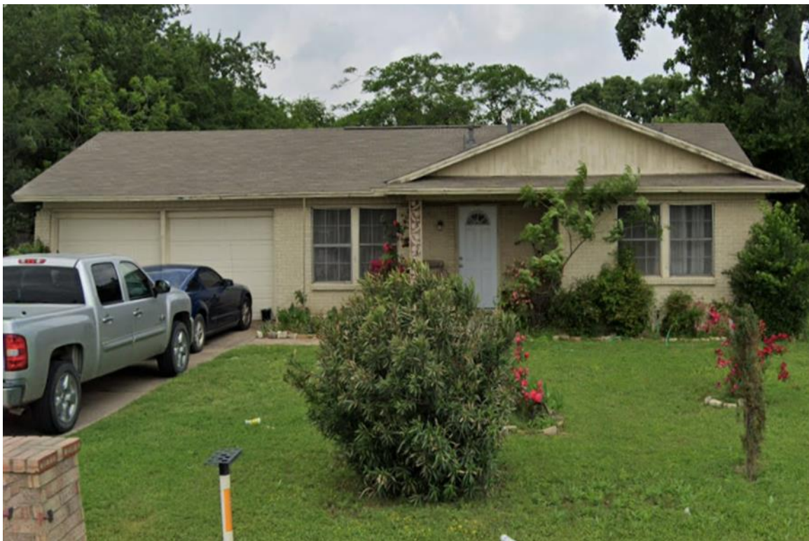
View of front elevation, facing north (image courtesy of Google Streetscape, 2019)
