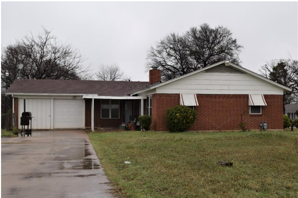
Facing north, view from the frontage road
