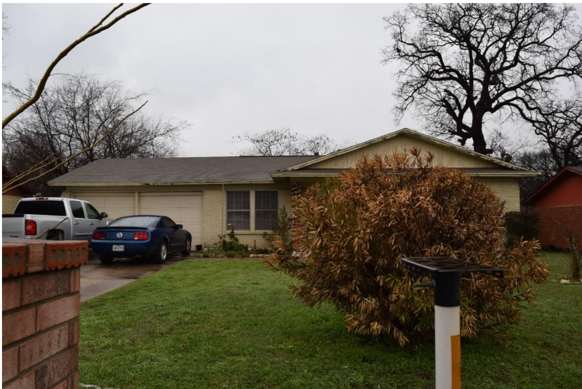
Front elevation, facing north
