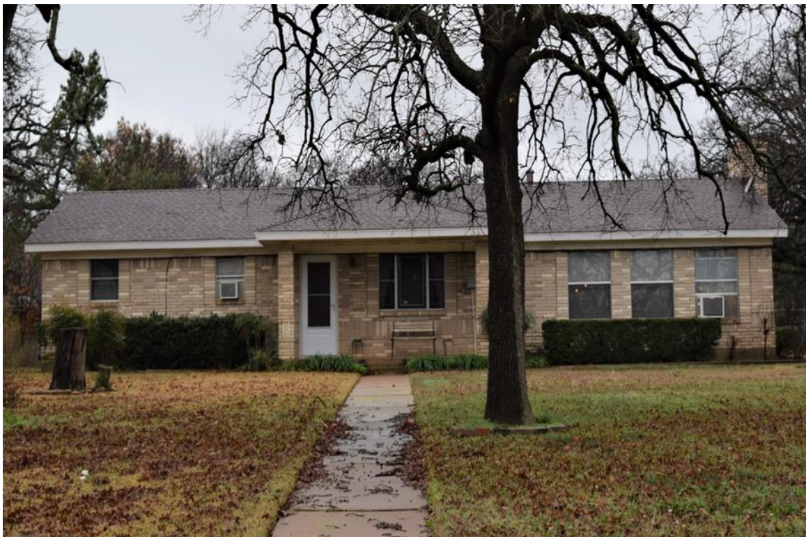
View of front elevation, facing west
