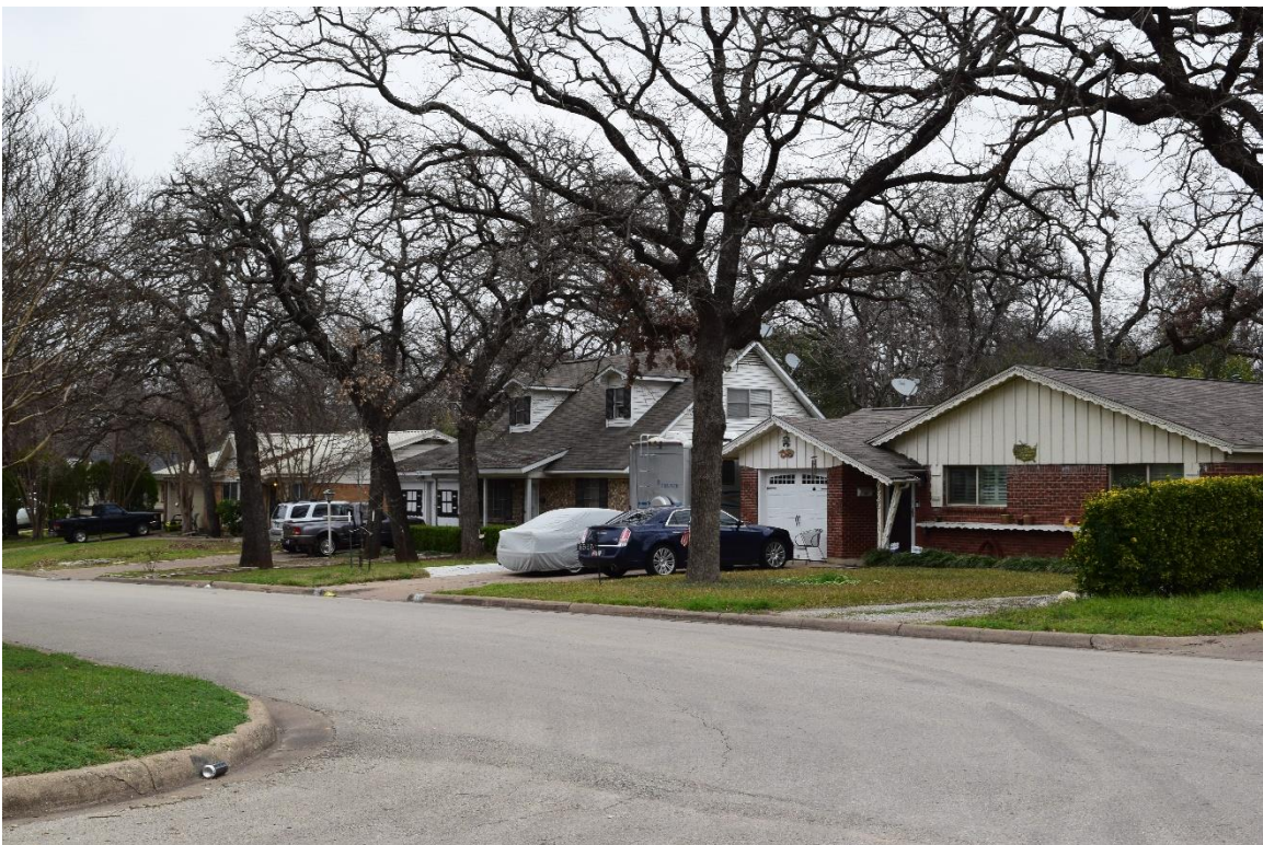
F25: Overview of residences on Shady Hill Drive East, facing northeast
