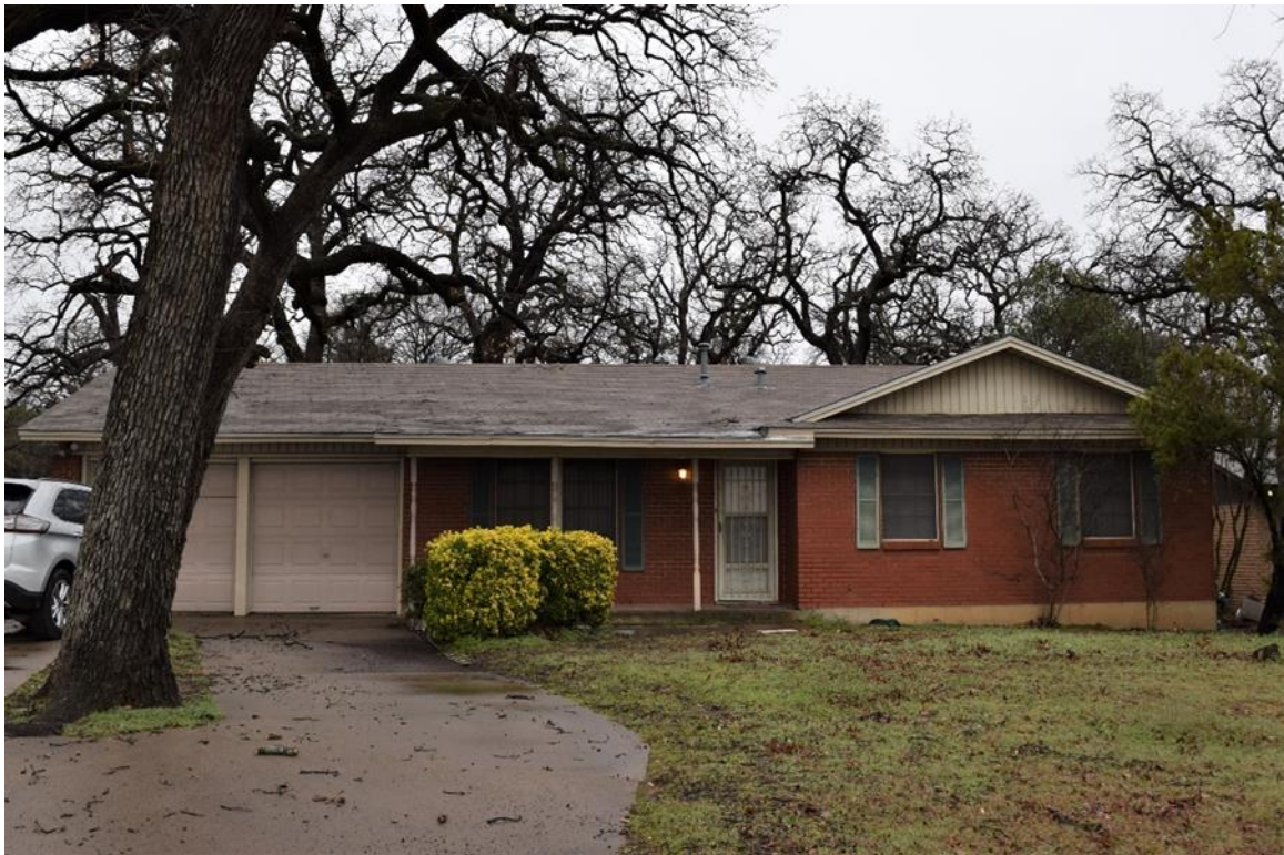
View of front elevation, facing north
